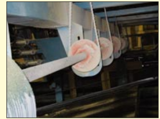
Sawmill Line Shaft Conveyor
